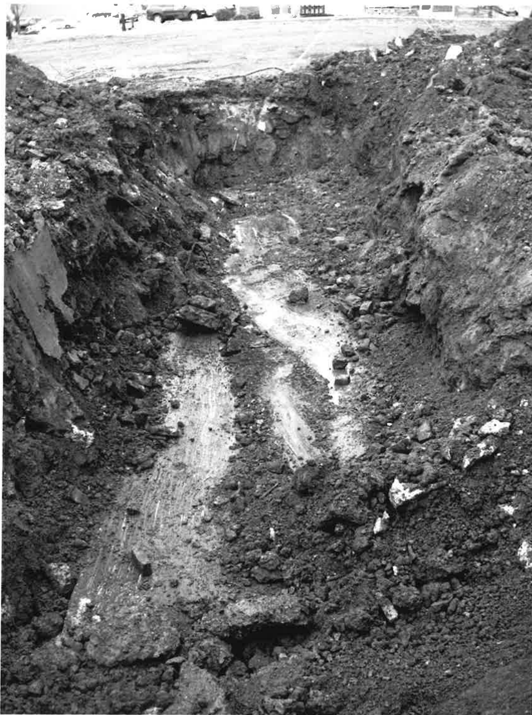
Figure 1. Concrete and brick encountered onsite to suggest concentrations at depth could be from application around historic foundations of the flourmill site.
