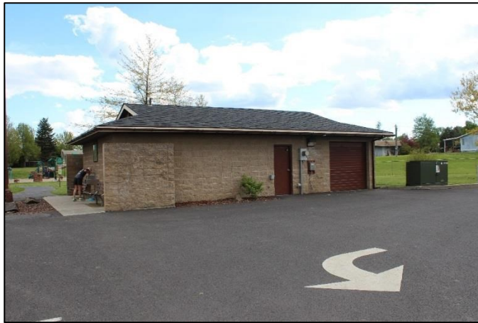
Bathroom facility (new roof)
