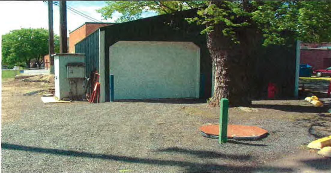
Front of building
