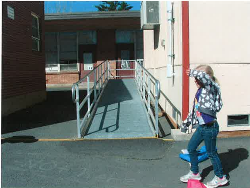
Picture taken 4-09-2013 – West Park Elementary Additional Modular Classroom Southeast Corner -South Face of Classroom Lowest Adjacent Grade- lowest machinery – lowest stair support.
