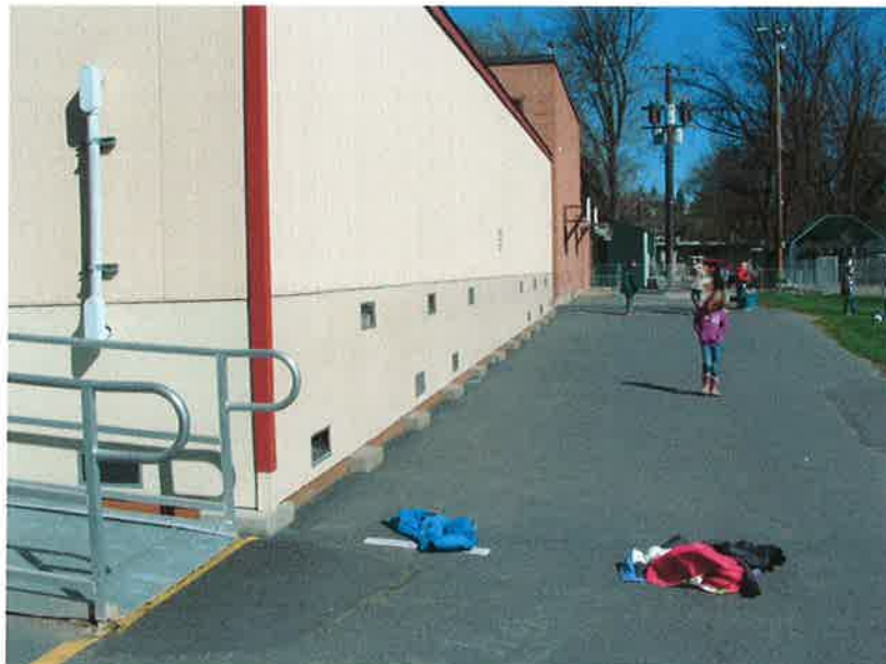
Picture taken 4-09-2013 – West Park Elementary Additional Modular Classroom Southeast Corner -East Face of Classroom Lowest Adjacent Grade- lowest machinery – lowest stair support.
