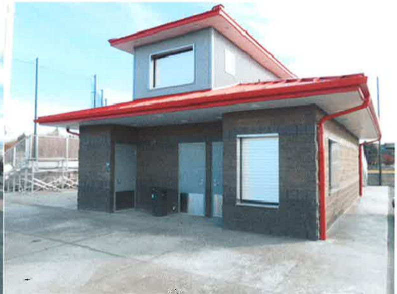
Northside of building with restroom, upstairs, and concession stand access. West face concession access.
