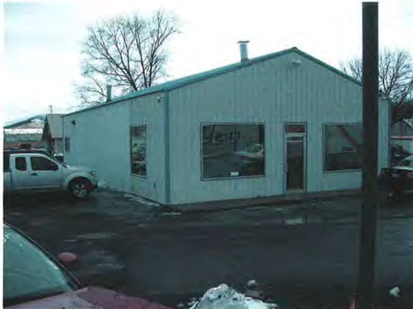
Existing Building without new addition Street View / West Face Picture Taken 12-16-09
